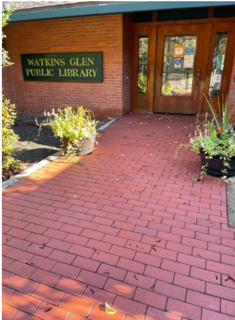
Watkins Glen Public Library in Schuyler County, New York. Improved accessibility project that features ADA compliant sidewalk entryways.
